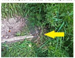
A broken riser on the steps at the bottom of Church Field
