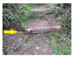
In the absence of any likely action by Essex CC, the step riser has been replaced and secured and the step infilled.
