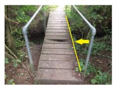
The defective plank on the bridge partially collapsed and the support beam (underneath the yellow line shown above) appears to have broken.
