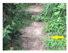
The step riser collapsed completely.
