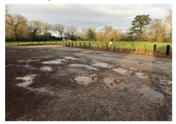
Although most of the deepest potholes have now been temporarily filled, it is evident that 'make-doand-mend' attempts to maintain and repair the surface do not provide a suitable long-term fix.
