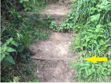
The step riser collapsed completely.
