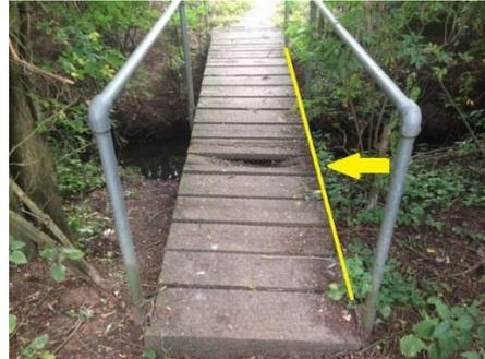
The defective plank on the bridge partially collapsed and the support beam (underneath the yellow line shown above) appears to have broken.
