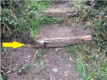
In the absence of any likely action by Essex CC, the step riser has been replaced and secured and the step infilled.
