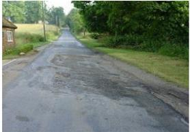
That has meant an on-going problem with verge erosion and water and sediment flowing down the hill during heavy rainfall, strewn stones and debris across the road.
